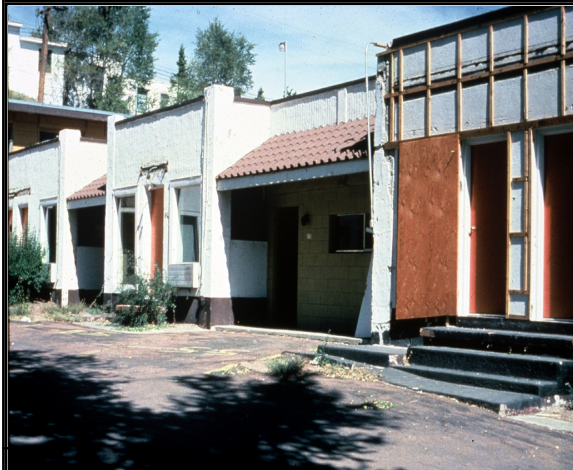
Abandoned Motel after Colorado Avenue ceased being US 24 West.
